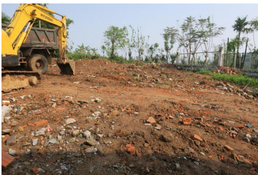
Construction begins on the Cu Ty Kindergarten- Quảng Trị Province
