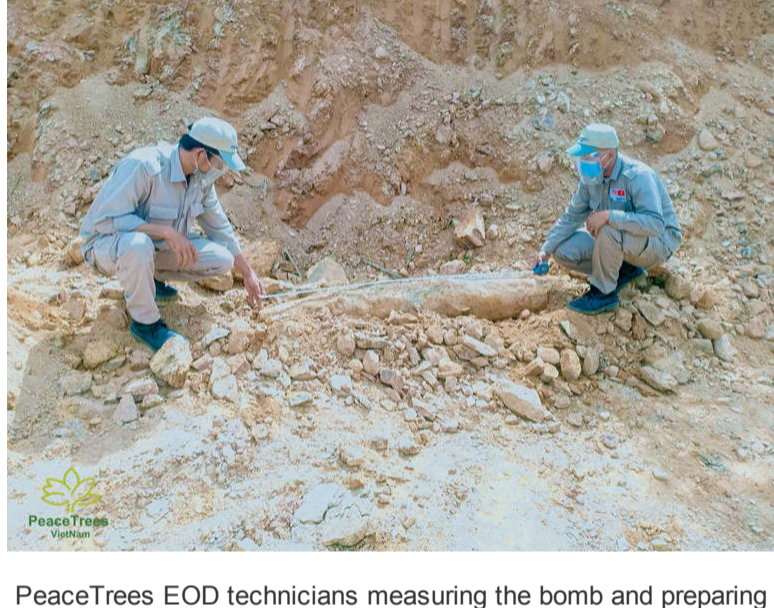
PeaceTrees EOD technicians measuring the bomb and preparing it for removal
