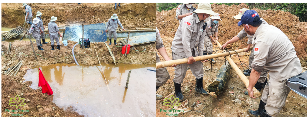
A PeaceTrees EOD team pumping water out of the channel to access the bomb, Dong Hoi City, Quảng Bình Province
