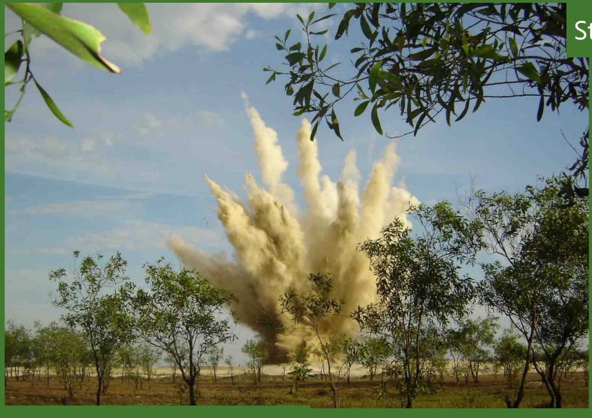
Demolition blast at grand demolition site in Hai Ba, Hai Lang
