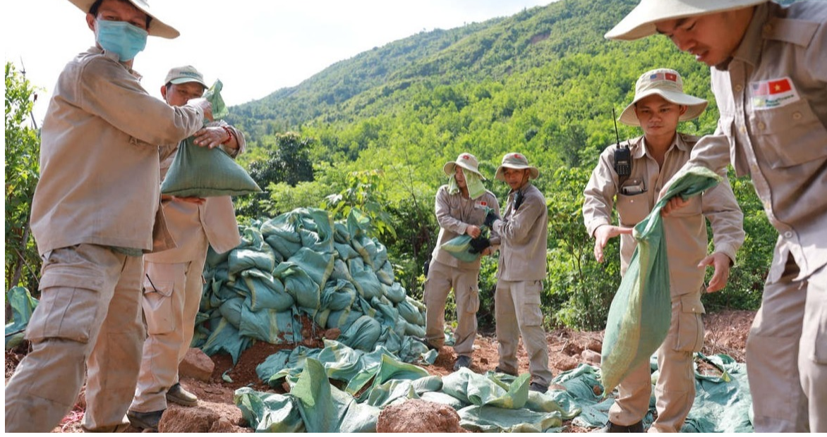
PeaceTrees deminers lining up sand bags at the demolition site to minimize the damage of the planned explosion- June 2, 2021
