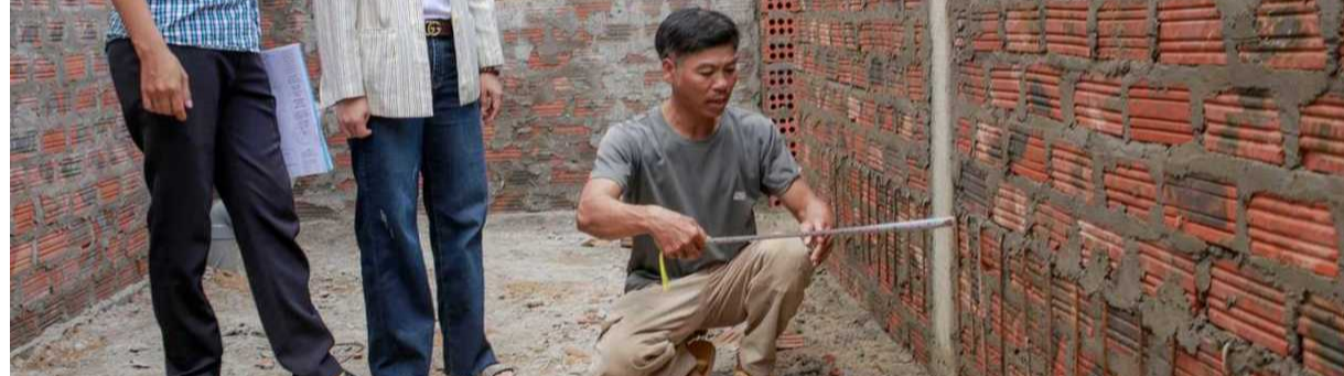
Prin Thanh Kindergarten construction in progress - May 2020
