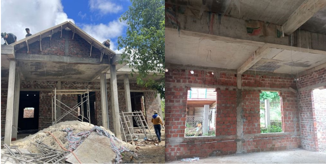
Construction workers at the CuTy kindergarten- Quảng Trị Province
