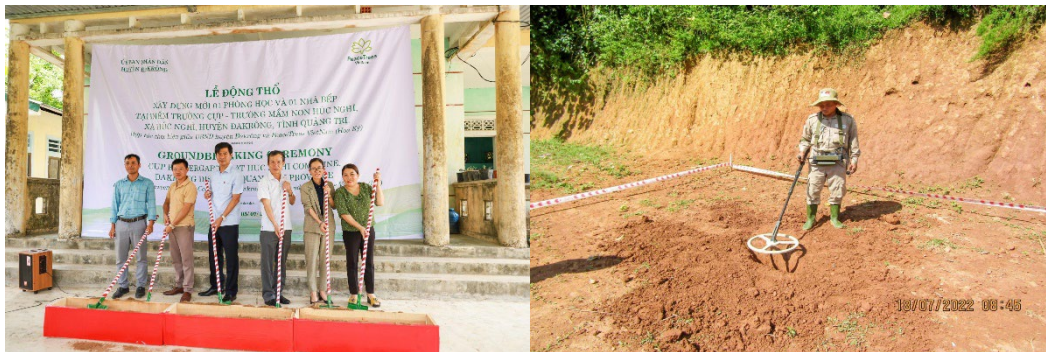
PeaceTrees Vietnam in-country staff and partners at the groundbreaking ceremony- Quảng Trị Province
