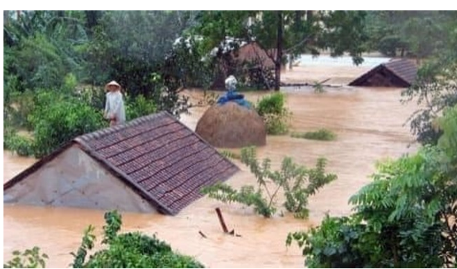
Flood waters have risen up the roof tops in some parts of Central Vietnam.
