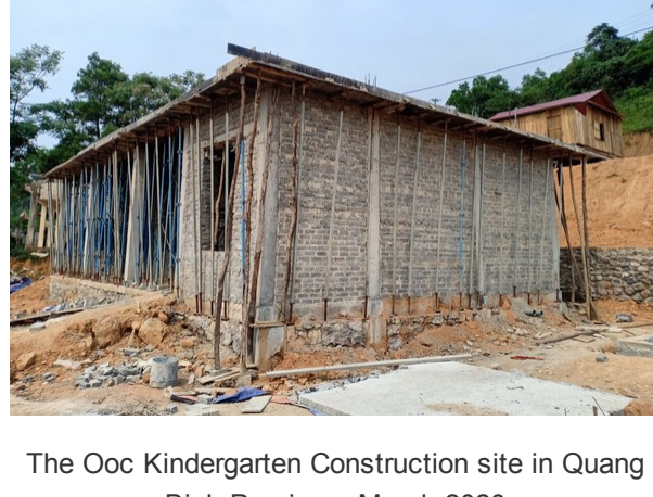
The Ooc Kindergarten Construction site in Quang Binh Province- March 2020
