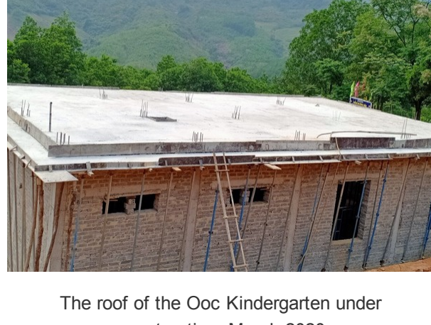
The roof of the Ooc Kindergarten under construction- March 2020
